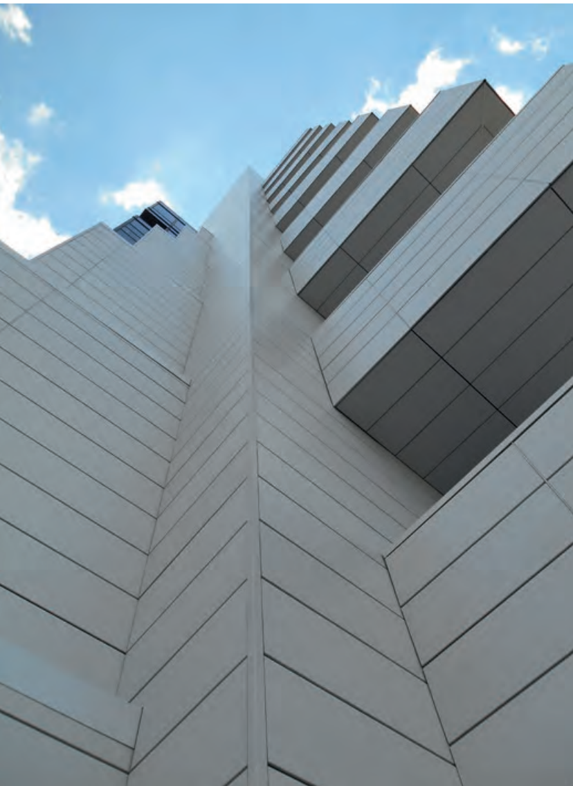
The new building shell
