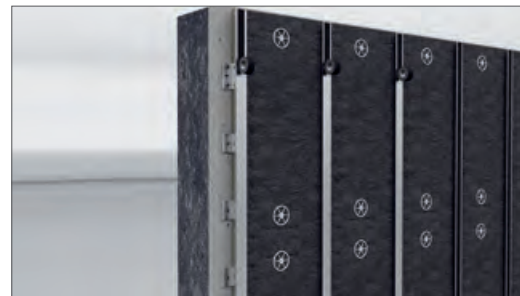
Apply joint tape on vertical bearing profiles
