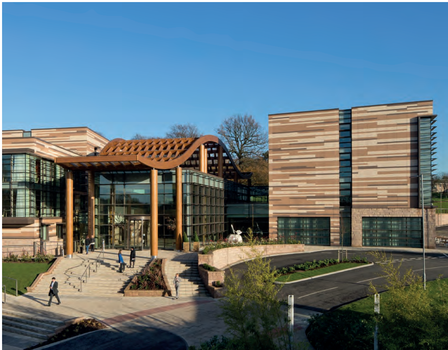
Orchard Hotel, Nottingham, Great Britain / RHWL Architects Ivory House, St. Katharine Dock, London / Completion: 2012
